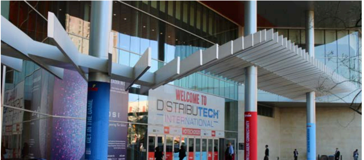
MAIN LOBBY EXTERIOR WINDOWS, DOORS, AND COLUMNS
